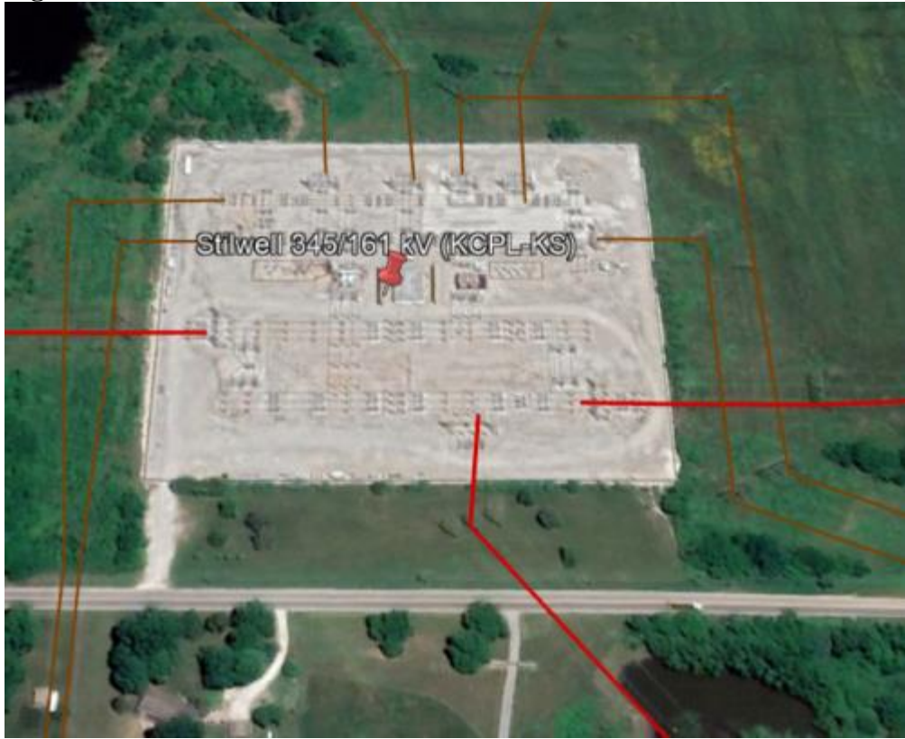
Figure 28 – Stilwell 345 kV substation
